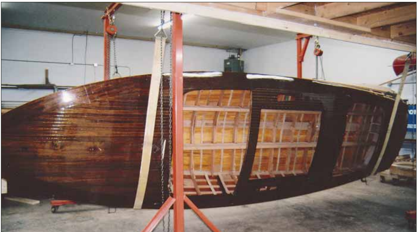
Once the new bottom is installed, the boat can be turned over so work can begin on the decks.
